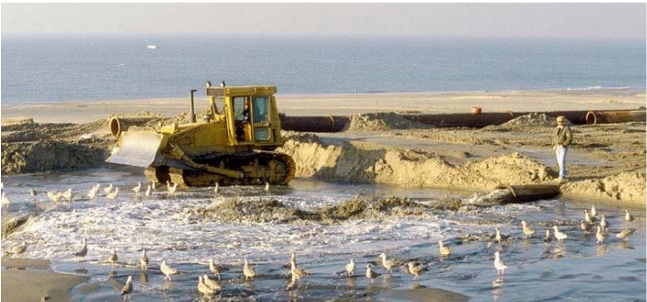
Figure 10: Beach nourishment on the Dutch Wadden Sea island Texel. Source: Ecomare. Copyright Sytske Dijkse.
