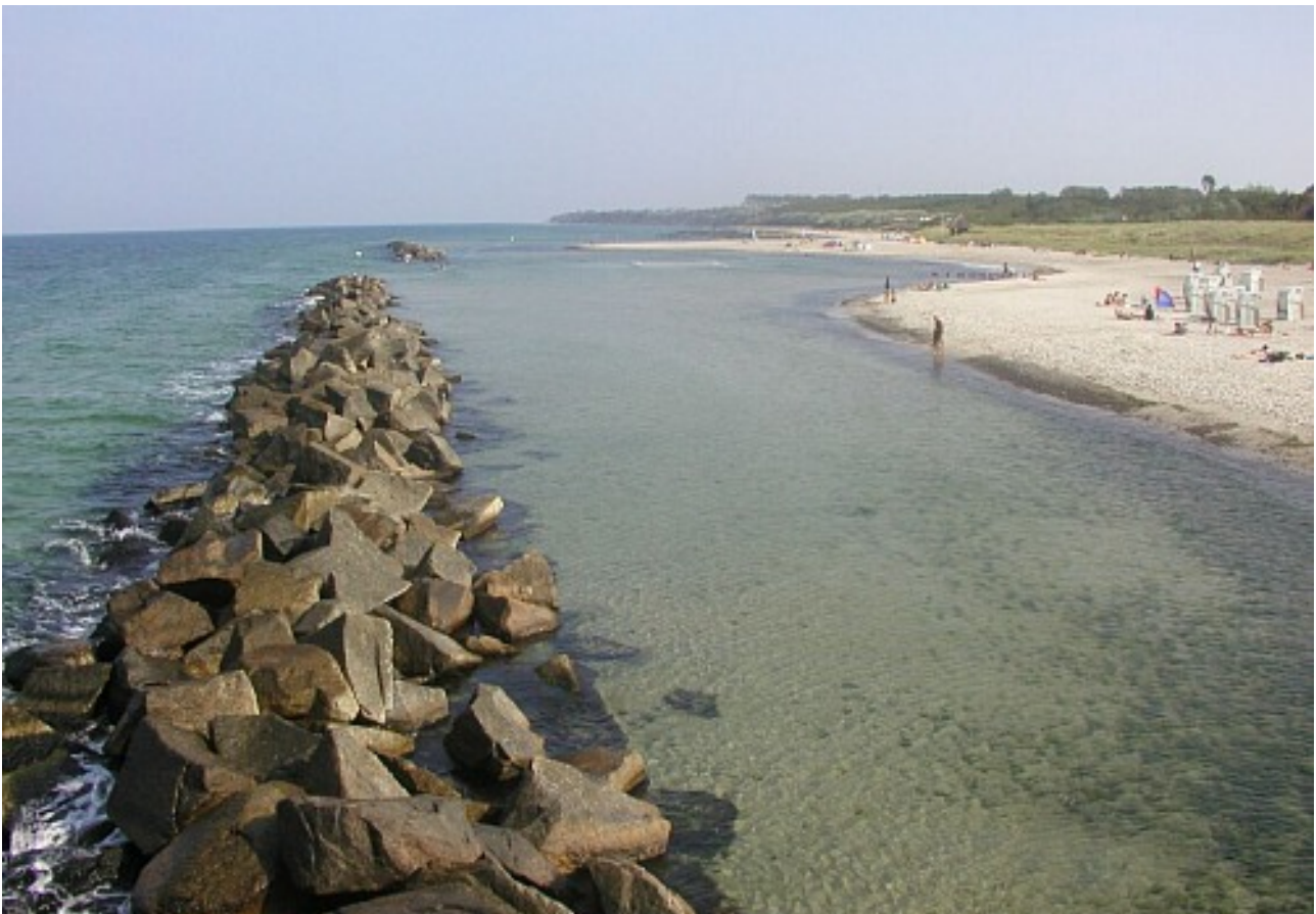
Figure 6: Breakwaters in front of a public beach.
