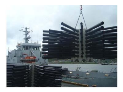
The cylinder is filled with stones to increase weight and stability. From the cylinder 14 vertical rows of 2.5m long polyethylene pipes – with a diameter of between 9 and 18 cm – radiate outwards. Together, the cylinder and plastic pipes on each unit provide an external and internal surface area of  $250m^2$ , the pipes provide 300m pipe length, and the total weight is 9 metric tonnes.
